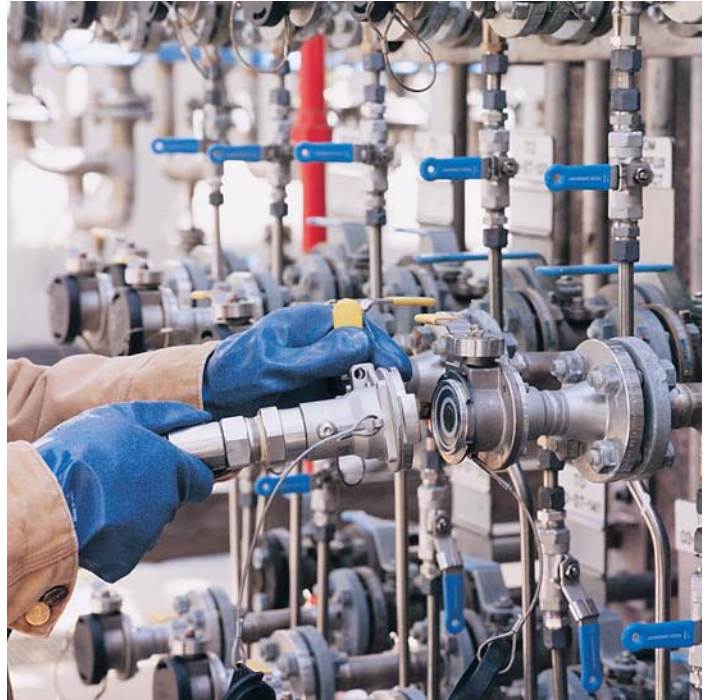
Manifold station with EPSILON® adapters.
